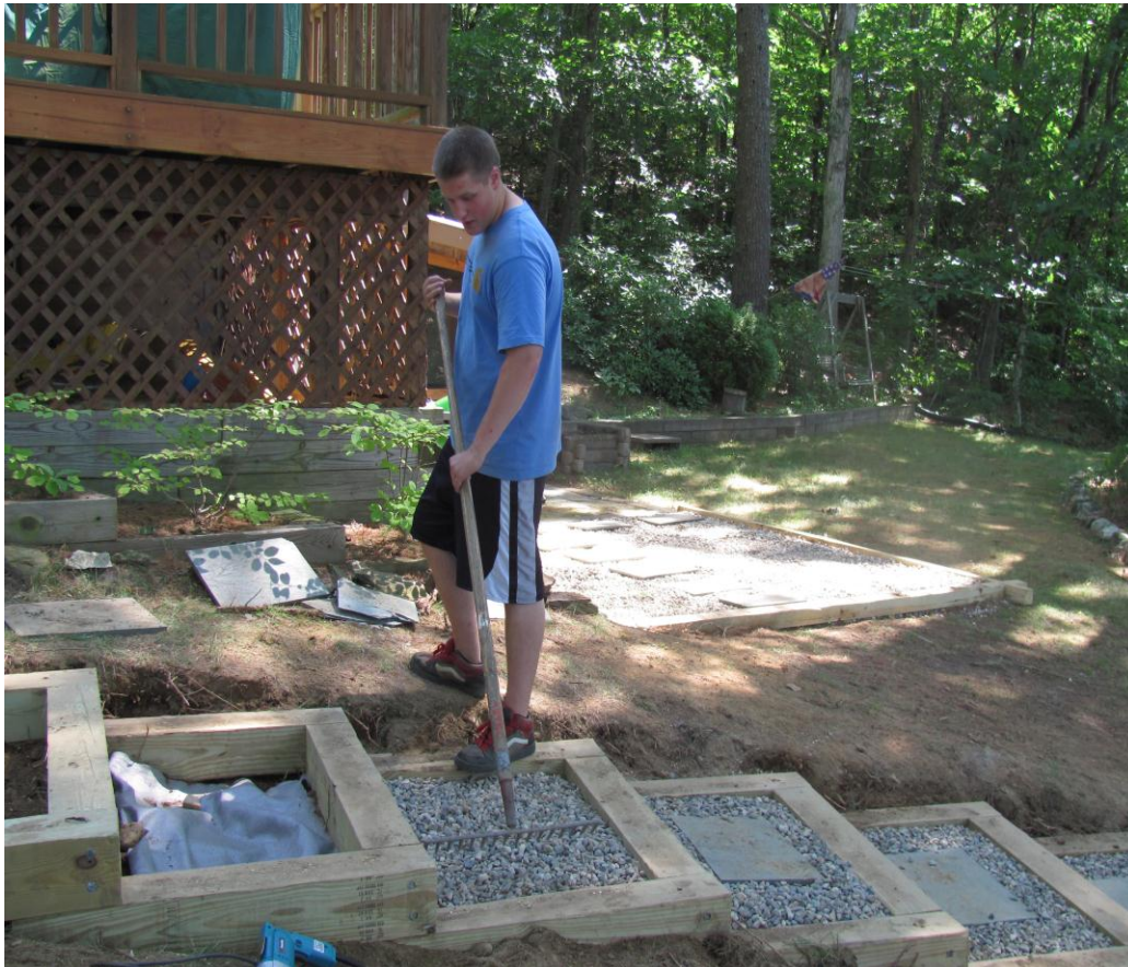
2 -An ECC member working on infiltration steps
