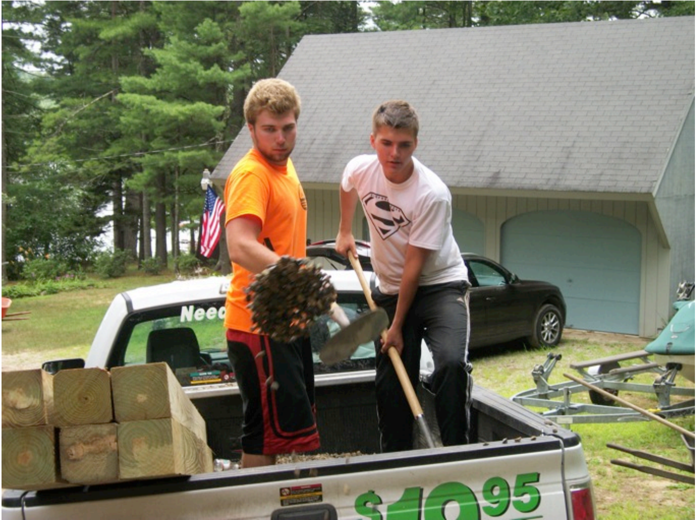
Photo 2013: Erosion Control Crew
