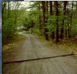
Rubber Razors direct water off the driveway or road and into vegetation with rubber razors.
