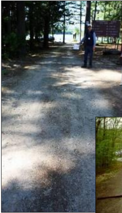
Rubber Razors direct water off the driveway or road and into vegetation with rubber razors.
