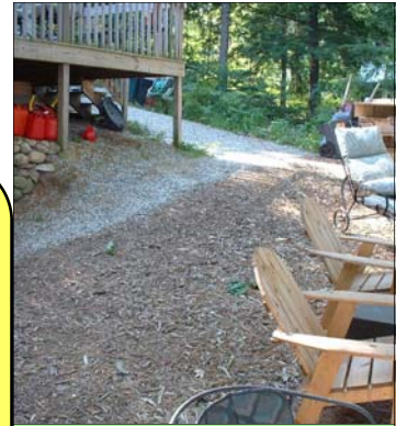
Mulch —Place mulch such as P&K Gravel's "fine erosion control mix" on bare soil.
