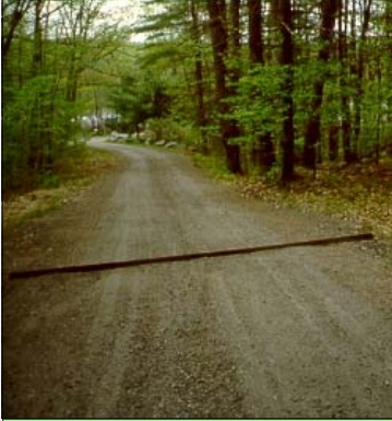
Rubber Razors —Direct water off the driveway and into vegetation with rubber razors.
