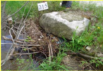
Problem — Culvert clogged with debris Solution — Remove debris and regularly inspect culverts to ensure proper functioning
