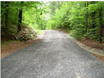
Road Material — Add hard-packing, cohesive surface material to the driveway.
