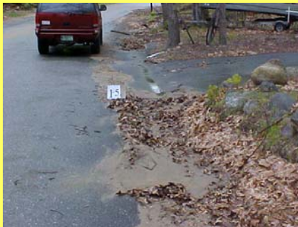
Problem — Inadequate ditching with erosion and sediment accumulation Solution — Reshape ditch, clean out sediment, vegetate, and install check dams
